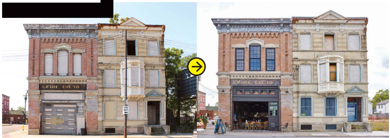
SLOW BURN Fireside Pizza opened in September 2014, in an historic firehouse barely saved from the wrecking ball.
